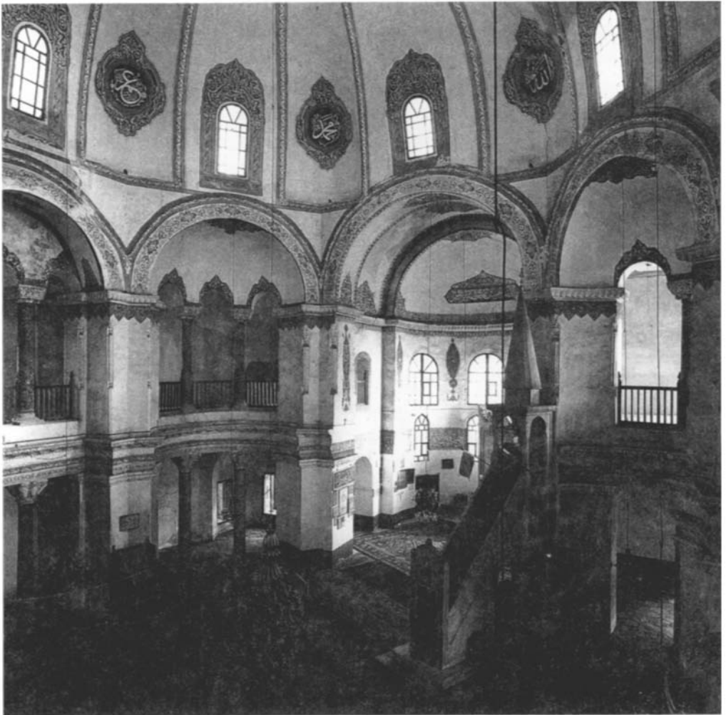
The interior of Ss. Sergius and Bacchus in Constantinople, built in 525, in which Justinian's architects attempted to solve the problem of superimposing a dome on a rectangular building. Courtesy of Josephine Powell, Rome.
